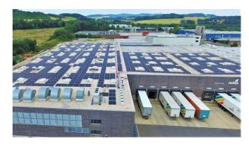
With the installation of more than 2000 photovoltaic modules at the Vlotho-Exter site in 2021, more than 160 single-family homes with 4 people each could be supplied for 1 year. The peak power is enough to cook lunch on 750 electric cookers. The generator area is 3,747 m<sup>2</sup>, which is about half a football field.
