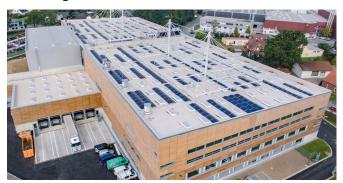
With the photovoltaic systems already in place on buildings B1 and B7 in Kirchlengern, the PV system on B7 has been extended by a further 230 kWp. The installation of 4,880 modules on the new multifunctional hall C3 in Kirchlengern is another example of our efforts to further advance the topic of renewable energies.
